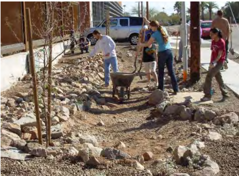
Rock edging along swale edges prevents erosion.
